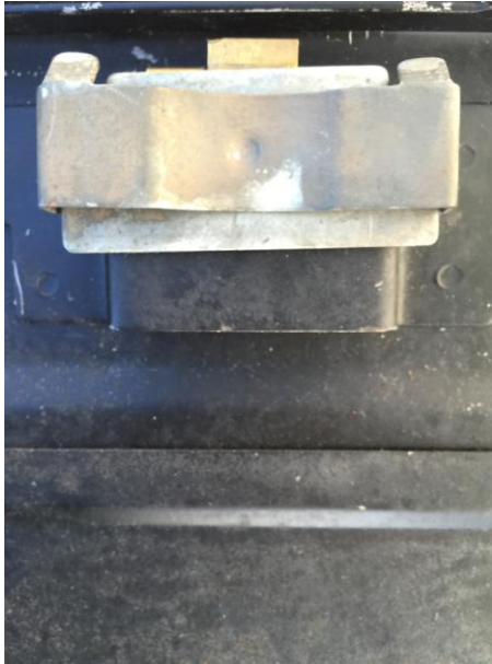
Inside of door - (bolt is thrown)
