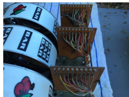
Wiring in reel assembly
