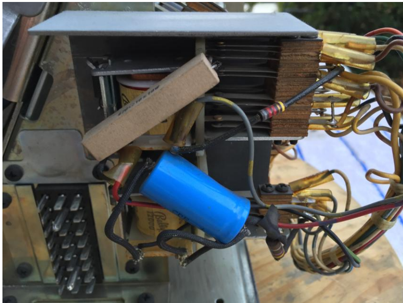
A wire wound resistor (tan, 10-watt) with two carbon resistors (in front of the relays); located on the hopper
